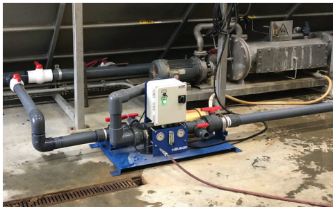
Moleaer's Nanobubble Generator integrates seamlessly into existing DAF.
